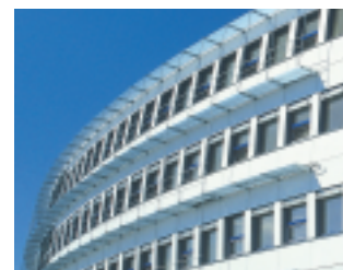
ENERGON Ulm: The admini- stration building of the Soft- ware AG foundation is the largest office building in the world built to the passive house standard. Thermix® warm-edge spacers are built into the windows and the facade.
